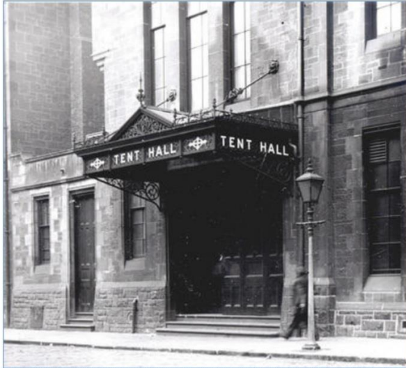
Tent Hall in Steel Street, possibly in the 1920s.
